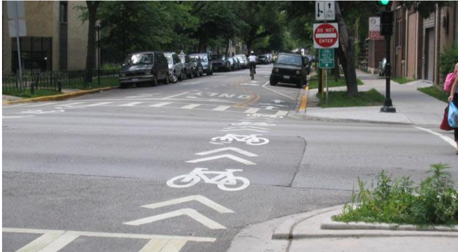
Figure 38. Pavement Markings through Intersections
