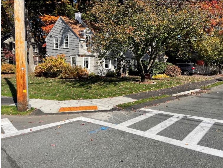
Figure 37. High Visibility Crosswalk
